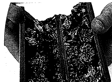
Pipe clogged with zebra mussels
